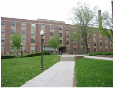
Figure 6. Typical Campus Bldg.
