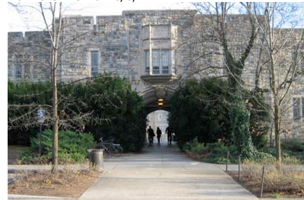
Figure 10. Norris Hall Breezeway
